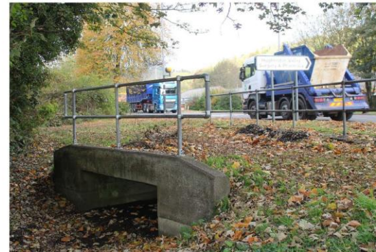
PHOTO 2. Side view SED 1 – Culvert Crossing
